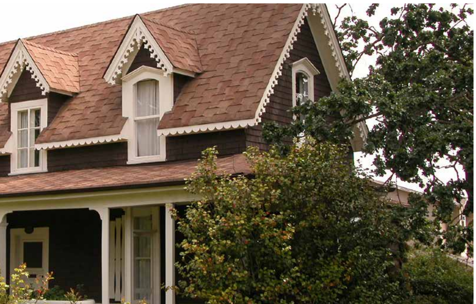
Heritage House, 3501 Cedar Hill Rd
